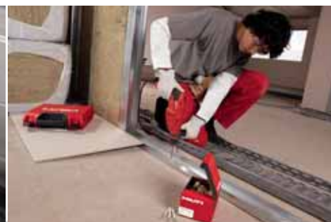
Drilling through drywall track into concrete.
