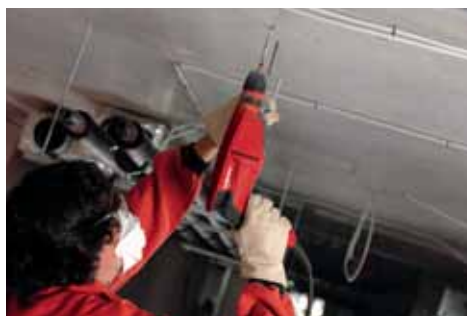
Anchor holes for plumbing, heating, ventilation and electrical installations.
